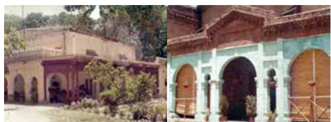
Residence of Hal (Rawalpindi Club)
