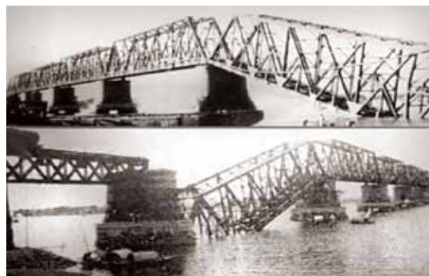
Meghna Bridge in erstwhile East Pakistan (1971 War) (Source: defence.pk)
