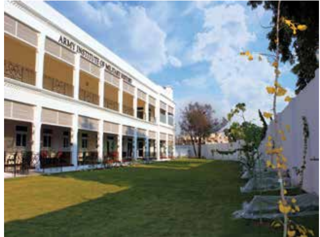
Newly constructed building of AIMH
