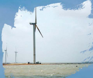
Foundation Wind Energy Limited I & II
