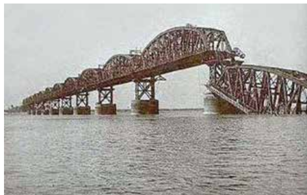
Hardinge Bridge after demolition (Source: bangladeshpost.net)
