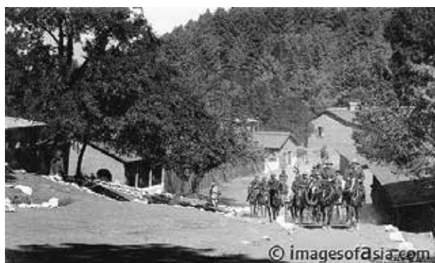
Royal Indian Army Service Corps School, Kuldana (Source: ivoanacom)
